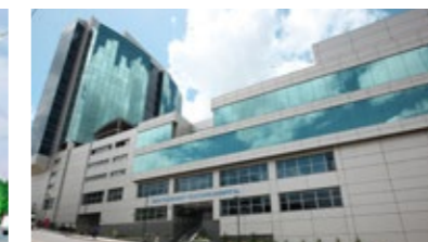
San Fernando Hospital Trinidad and Tobago
